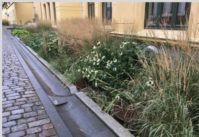
Figure 54, 55. Deichmans Gate and Wilses Gate, Oslo. Accumulation of rainwater in rain gardens and creating attractive features (water sculptures) at roof rainwater catchments. (photo by authors)
