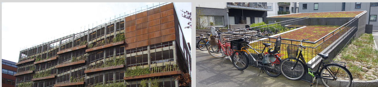
Figure 50, 51. The building complex makes extensive use of green facades (pictured here: a multi-storey car park) and green, extensive roofs with goldmoss coverings, which help collect rainwater and reduce roof overheating, improving the microclimate of the site (photo by authors)
