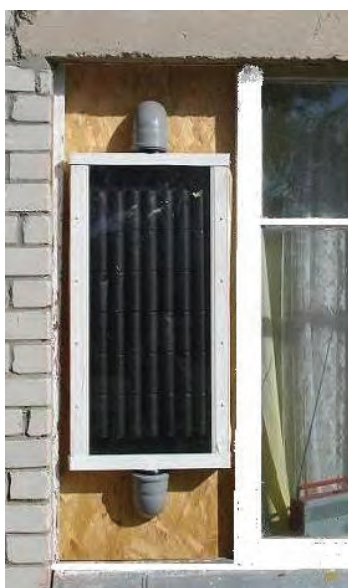
Figure 1. View of stationary solar collector with cylinders of black coloured cans situated on steel-tinsplate absorber.
