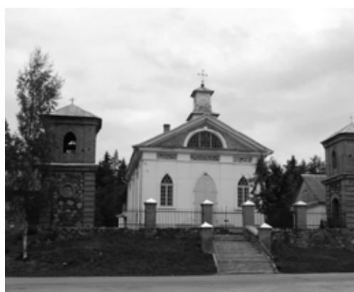
Figure 11. Free-standing bell tower in Borovka.
