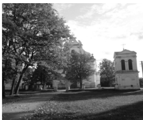
Figure 12. Free-standing bell tower in Šķaune.
