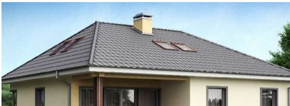
Figure 2. House roof under the construction.
