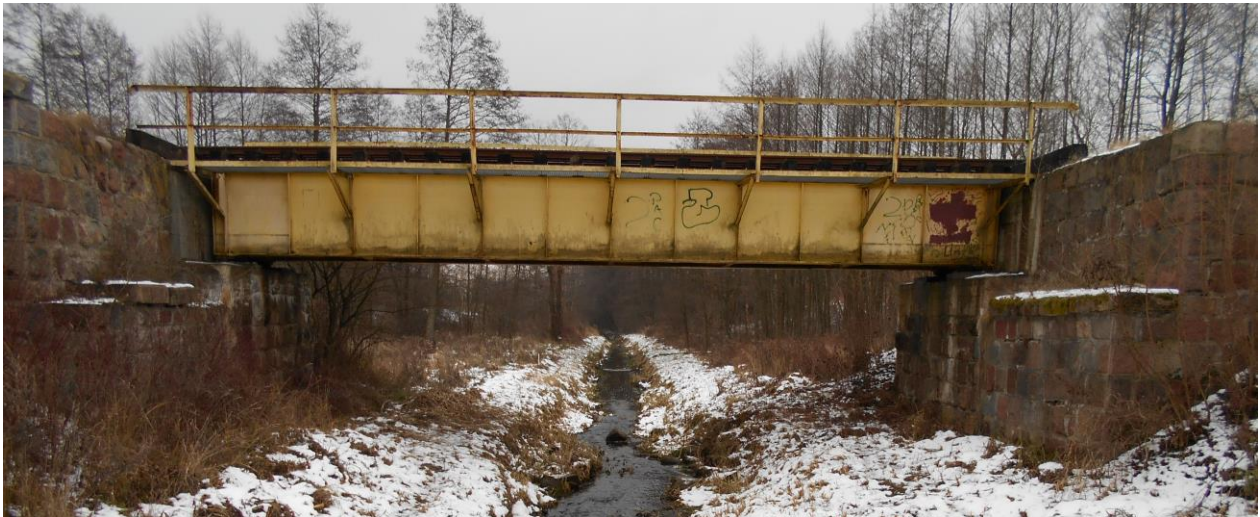
Figure 1. View of the bridge before disassembly.
