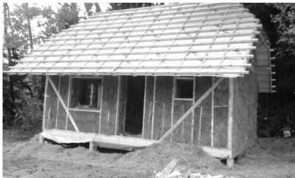
Fig. 4. External appearance of the sauna before rendering
