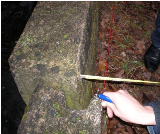
Figure. 2 Illustration of retaining walls deformations' measurements
