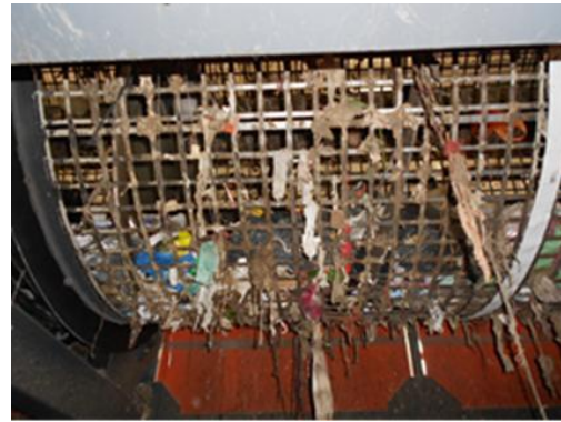
(a) The drum screen in Vibsteri (photo: Arina)
