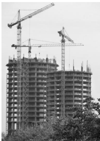
Figure 1. Multifunctional complex “Z-towers” construction process
