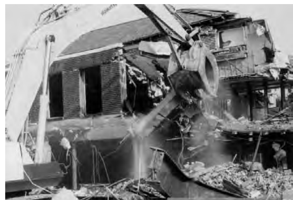
Figure 1. Demolition work of commissioned buildings.
