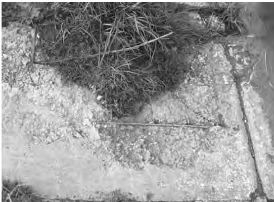
**Figure 2.** Erosion of surface on concrete slabs (Ageniskis pond) by influence of frost cycles.
