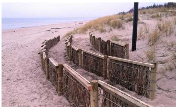
Fig. 1. Left: A sand catcher fence made of reeds, shortly after installation in the summer of 2018 near Carnikava. Right: The sand catcher fence has greatly increased the accumulation of sand [photographed in the autumn of 2019]
