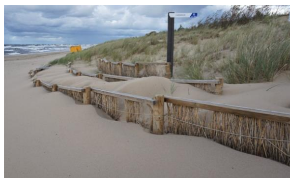
Fig. 1. Left: A sand catcher fence made of reeds, shortly after installation in the summer of 2018 near Carnikava. Right: The sand catcher fence has greatly increased the accumulation of sand [photographed in the autumn of 2019]
