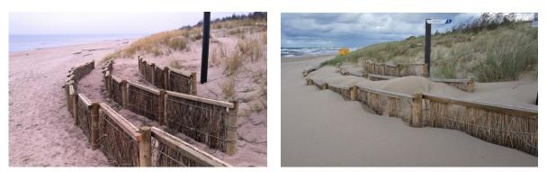
*Fig. 1. Left: A sand catcher fence made of reeds, shortly after installation in the summer of 2018 near Carnikava. Right: The sand catcher fence has greatly increased the accumulation of sand [photographed in the autumn of 2019]*
