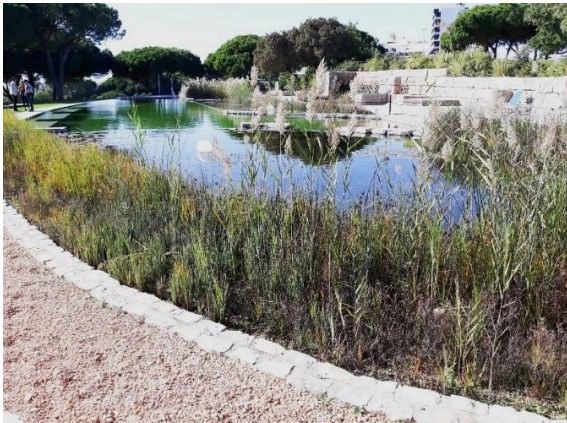
Fig. 6. A biophilic pool in Albufeira, Portugal, was designed for swimming in contact with nature while avoiding allergies from pool chemicals due to water purification using plants [photo: T. Panagopoulos]
