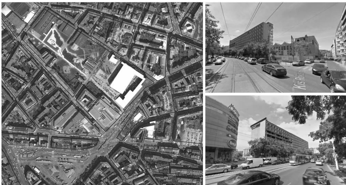
Fig. 3. Business as usual state with the existing ministry building and underutilised sites around it [google.com, just before the demolition]
