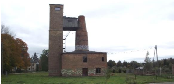
Fig. 7. Brick firing kiln in village Ceplis [Source: A. Katlapa]
