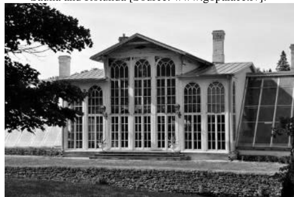
Fig. 19. Palmse Manor Palm House [Source: www.panoramio.com ].
