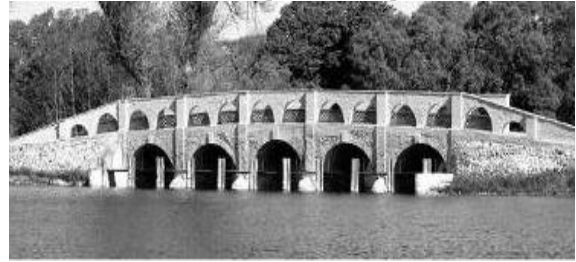
Fig. 39. The Original Arch Bridge [Source: www.pakruojistic.lt].
