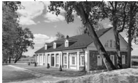
Fig. 14. Renovated Building of the Bistrampolis Manor complex [Source: www.bistrampolis.lt].
