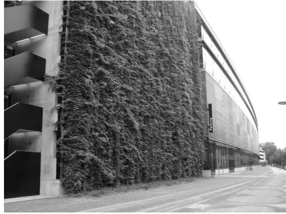
Fig. 4. Interaction of the building with vegetation following the mean “application”. Trade centre “Sihlcity”, Zurich [Source: photo by the author]
