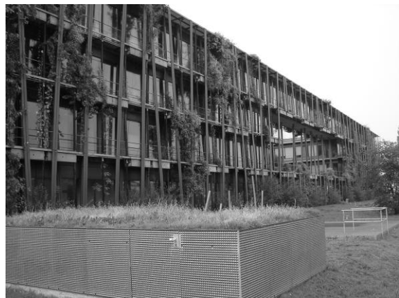
Fig. 5. Possibilities to introduce the containers with the plants in the structure of building facade. Walter Nernst-Haus, Institute of Chemistry, Humboldt University, Adlershof, Berlin, Germany [Source: photo by the author]
