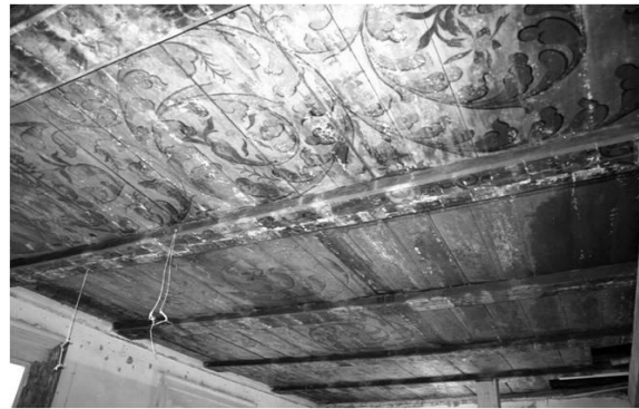
Fig. 8. ceiling paintings in the central room of the second floor. The mid-18th century (2006) [Source: photo by the author]
