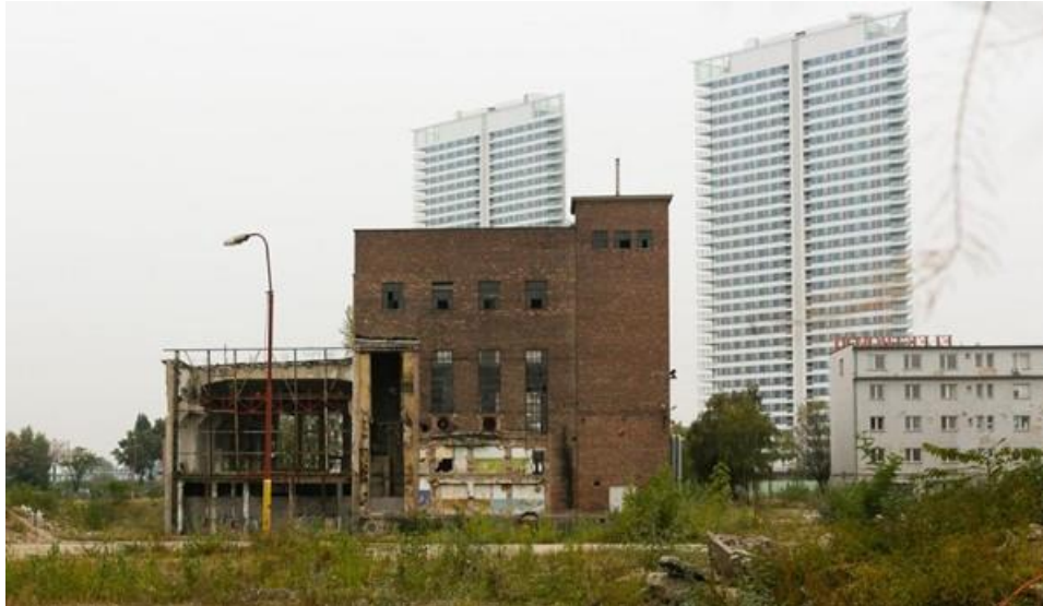
Fig. 5. The Jurkovic's heating plant
