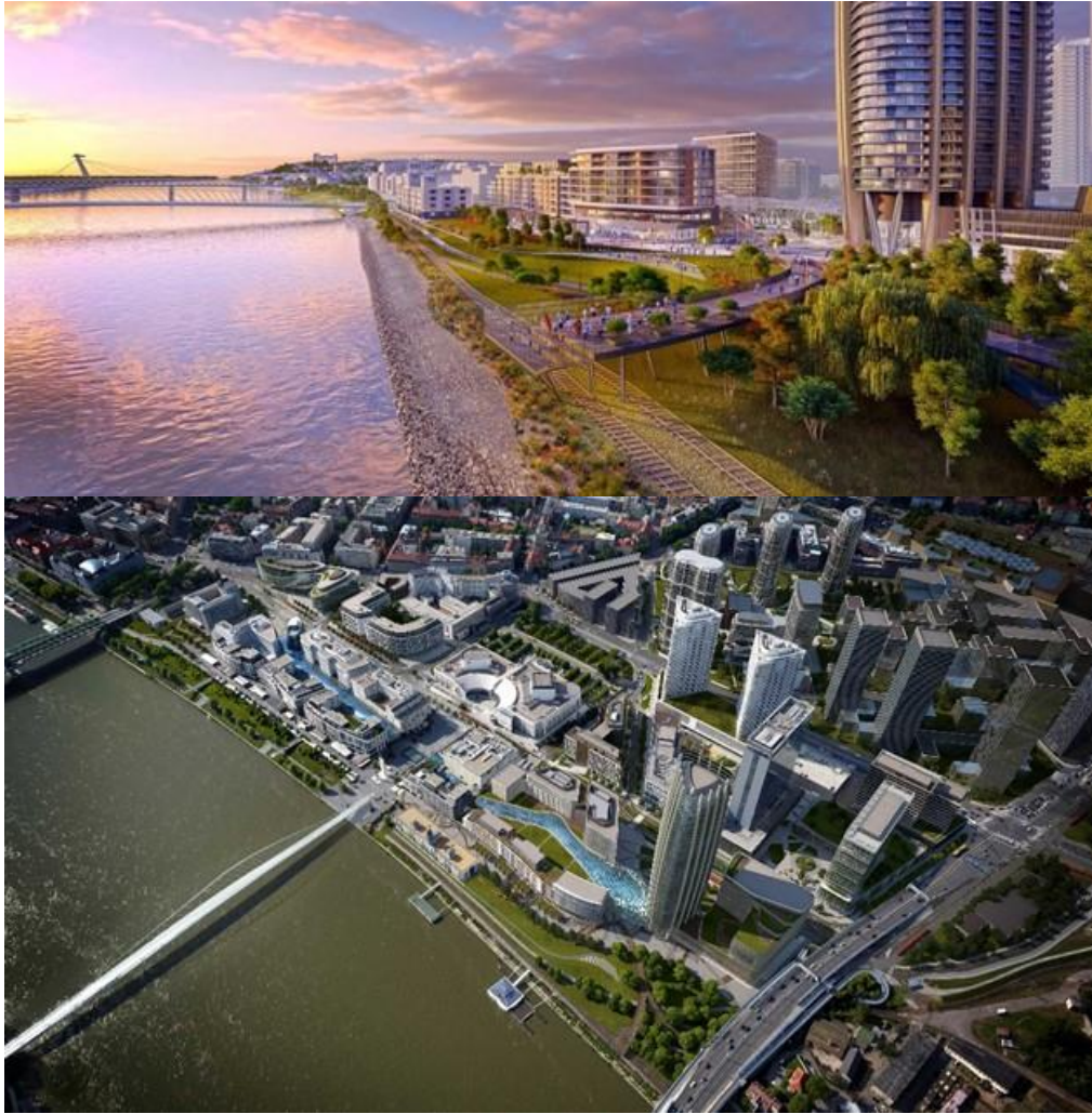
Fig. 9. The Eurovea and Eurovea II projects as a new city district Source: http://www.jtre.sk/projekty/eurovea-II
