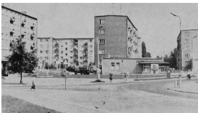
Fig. 3.5. Residential area in Jelgava in the second half of the 20th century [164, 172].
