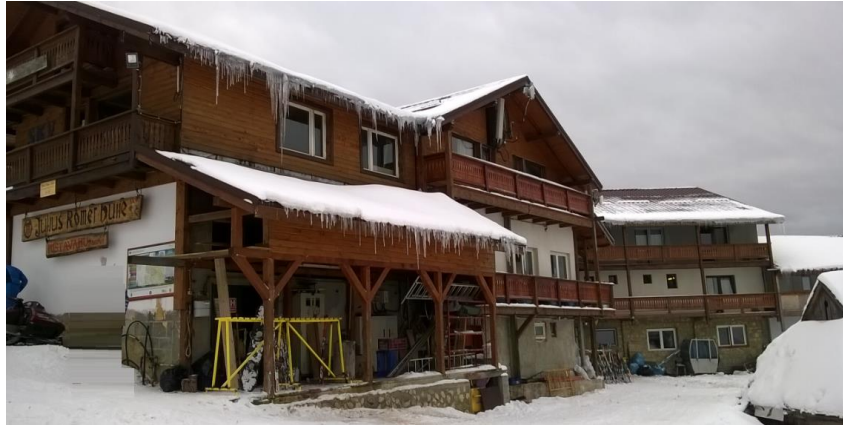
Fig. 1. The Postavaru Hut - Julius Romer Hutte
