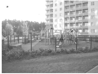
Figure 2.2. New area of dwelling houses with playground.
