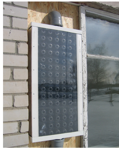
Figure 3. View of the solar collector with black polypropylene seed boxes absorber
