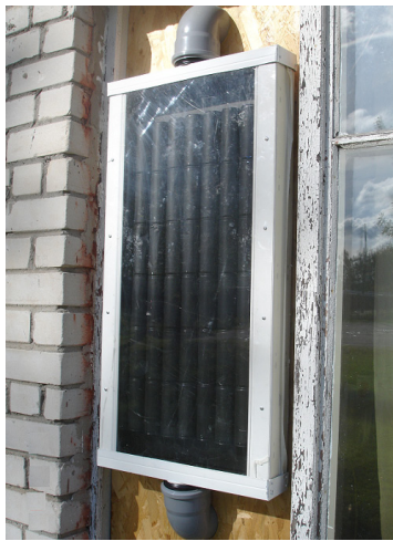
Figure 2. View of the solar collector with cylinders of black coloured energy drink cans situated on the steel-finplate absorber
