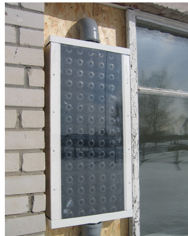
Figure 3. View of the solar collector with black polypropylene seed boxes absorber
