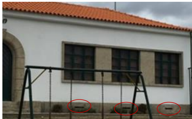
Figura 5 - Natural ventilation openings.
