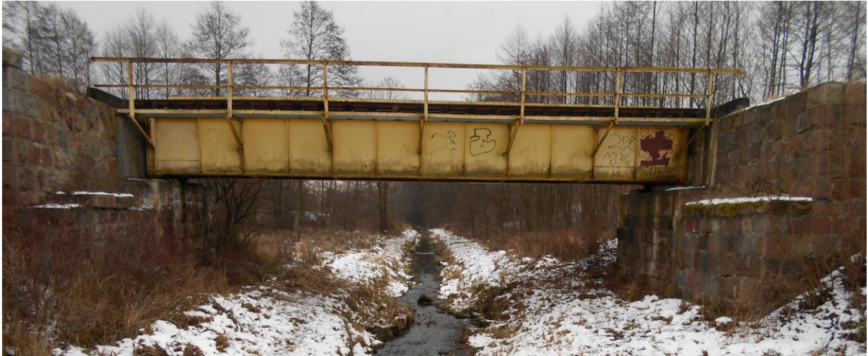
Figure 1. View of the bridge before disassembly.
