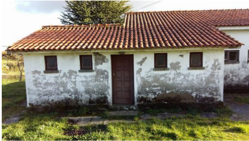
Figure 7 - Moss and painting's degradation
