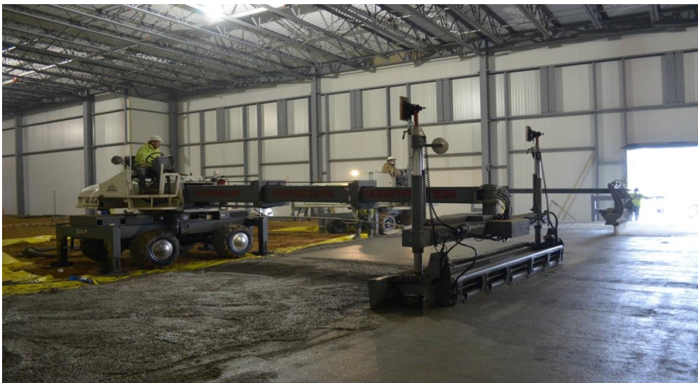
Fig.1 „Laserscreed” Insertion technology [16]
