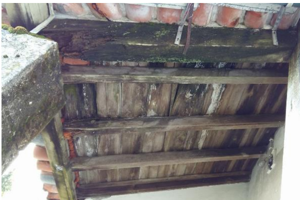
d) Rotting of the timber elements
