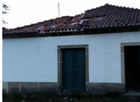
e) Absence and cracking of ceramic tiles
