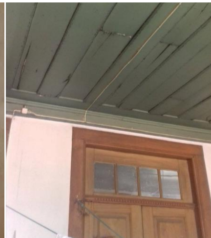
b) Timber ceiling and door
