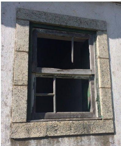
b) Rotting of the elements of wood
