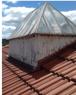
Figure 3 - Pitched roof with Marseille ceramic tiles and skylight
