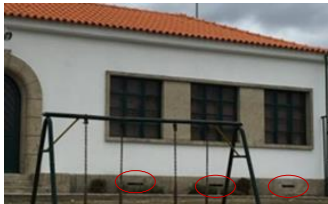
Figura 5 - Natural ventilation openings.
