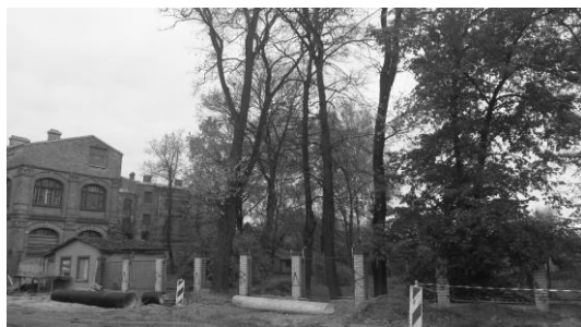
Figure 14. The tree group to the old Red Cross building to Driksa river (Source: photo by author, 2014)
