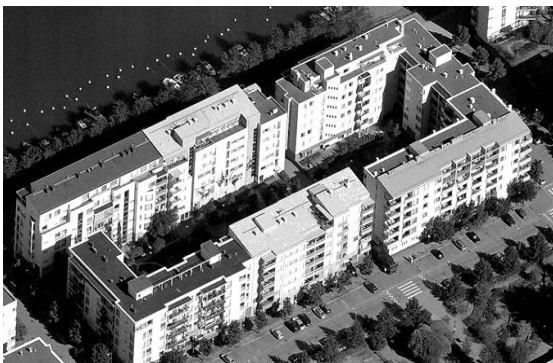
Figure 12. Residential area of Jatkasari, Helsinki (Source: http://www.bing.com/maps )
