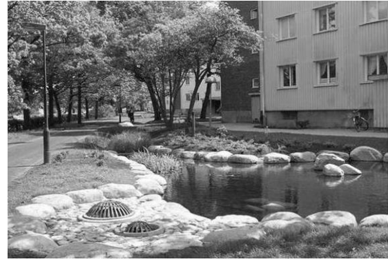
Figure 7. Designed shallow pond with rocky bed in Malmö, Sweden (Source: from project LV2003/005-876/VAPF/0029 materials)
