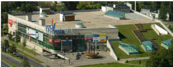
Figure 3. Green roof of the shopping centre Olympia (Source: www.bptam.com )
