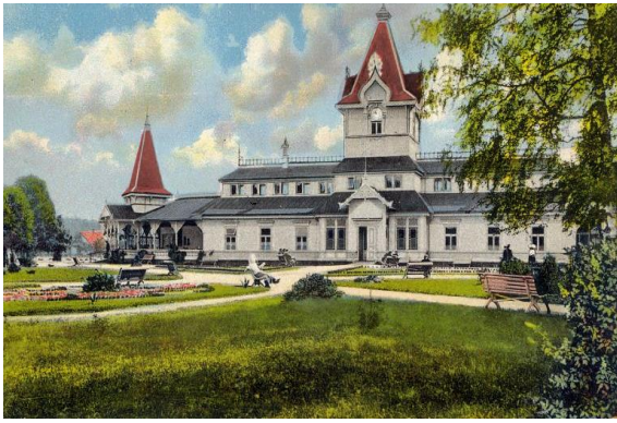
Fig. 10. The well-house plantations in the early 20 th century NKMP archive.
