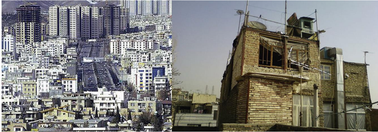
Fig. 3. An example of building regulation contravention in Tehran [14]
