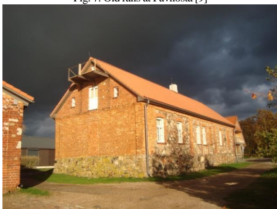
Fig. 8. The former pilot house [photo by the authors, 2017]
