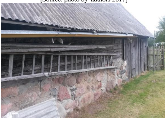
Fig. 12. Deep cattle shed at Sikrags [Source: photo by authors 2017]
