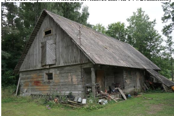
Fig. 7. An outhouse at Mazirbe [Source: photo by authors 2017]
