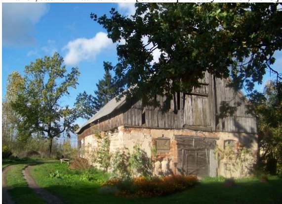
Fig. 8. Clay molding with stone joining elements in the corners. Jaunsvirlaukas Parish [Source: photo by author, 2013]
