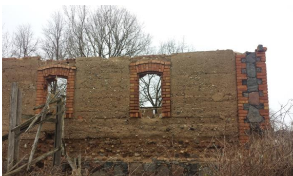
Fig. 9. The old cattle-shed has retained its rubble masonry, mortar finish, and the vertical plank pattern in the attic. Lestene Parish [Source: photo by author, 2013]
