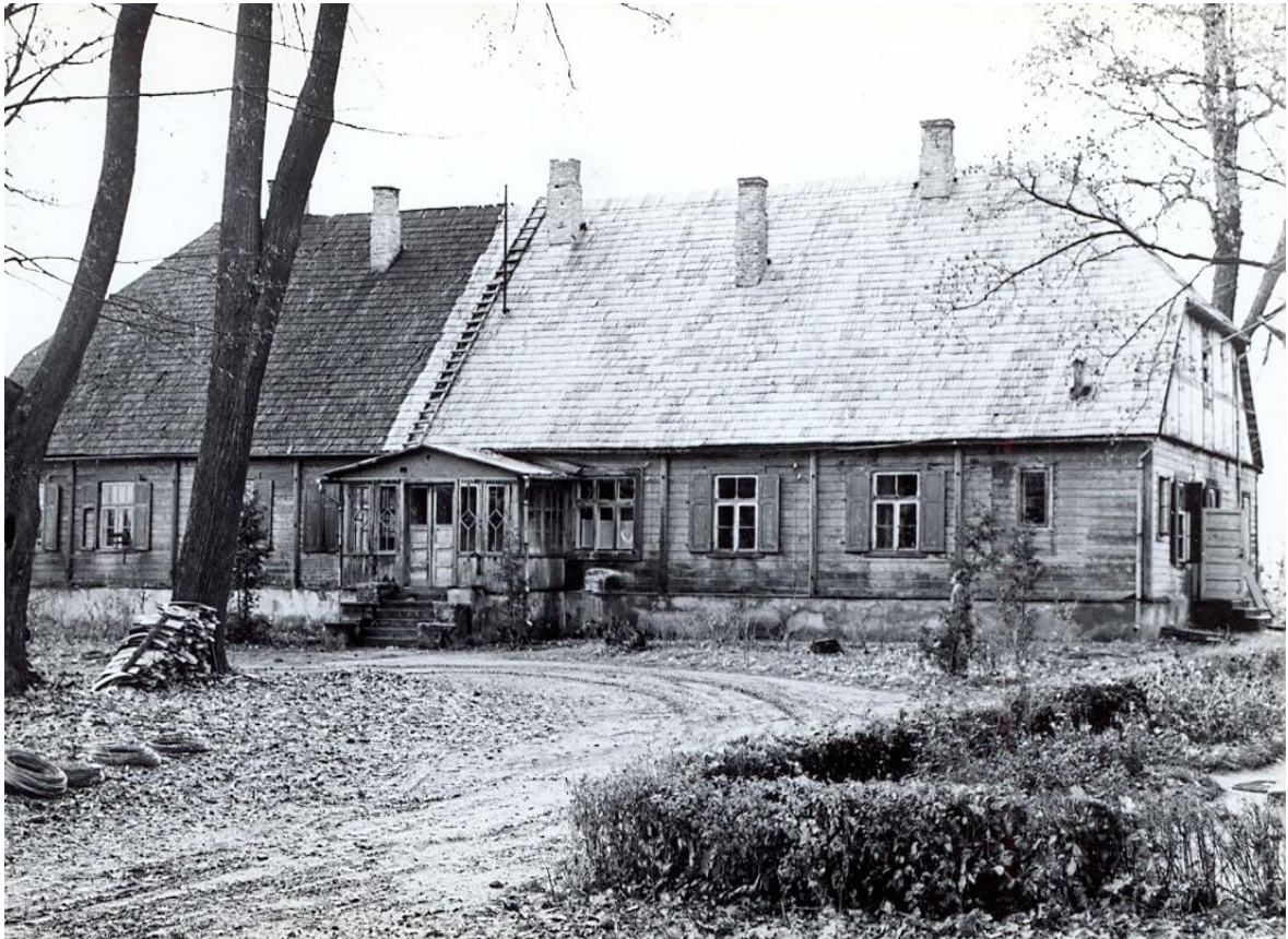
Fig. 2. The Valle pastor's house [Source: State Inspection for Heritage Protection of the Republic of Latvia, Monument Documentation Center, the 1960s]
