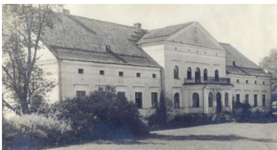
Fig. 1. The new manor house
