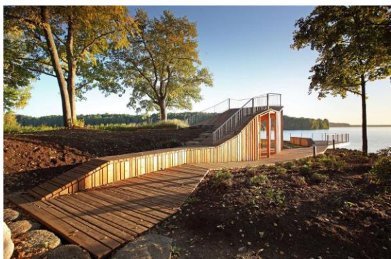
Fig. 28. The Observation platform and Pavilion [Source: http://www.designboom.com ]
