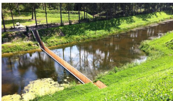
Fig. 29. The Moses Bridge - „Invisible Bridge” [Source: http://www.archdaily.com ]
