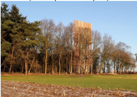
Fig. 3. Viewing tower at Vecht Riverbank [Source: http://www.archdaily.com ]
