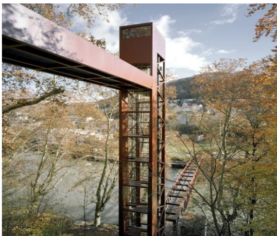
Fig. 30. Limmat Footbridge and Promenade Lift [Source: http://www.archdaily.com ]
