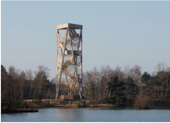
Fig. 1. The Lommel observation tower [Source: http://www.archdaily.com ]
