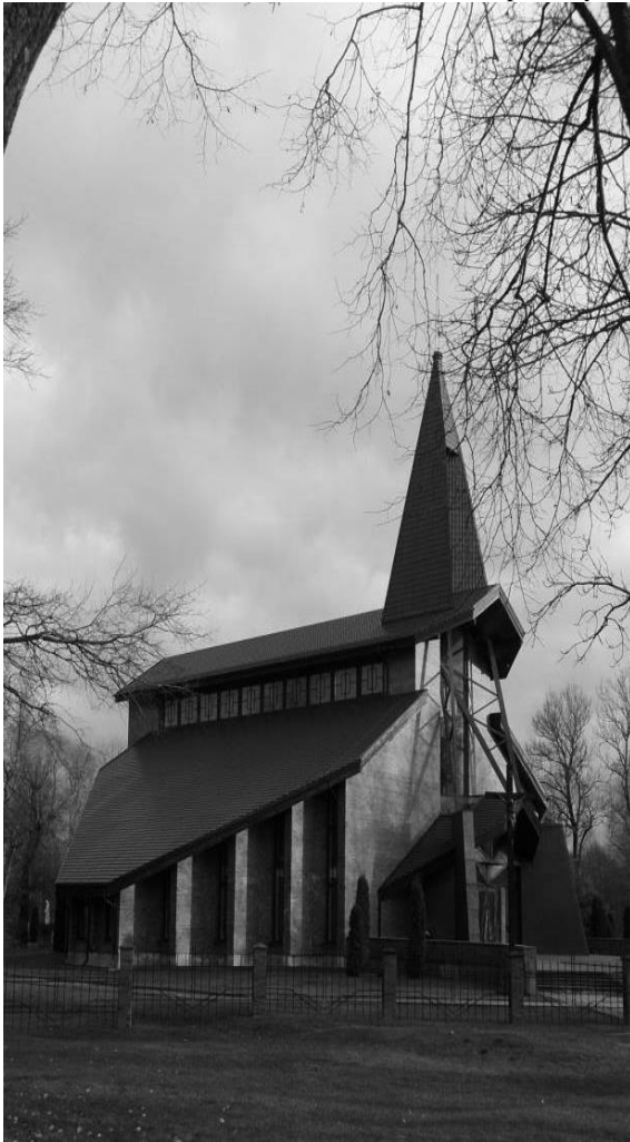
Fig. 5. Dobele Holy Trinity Roman Catholic Church, Baznīcas Street 10a
