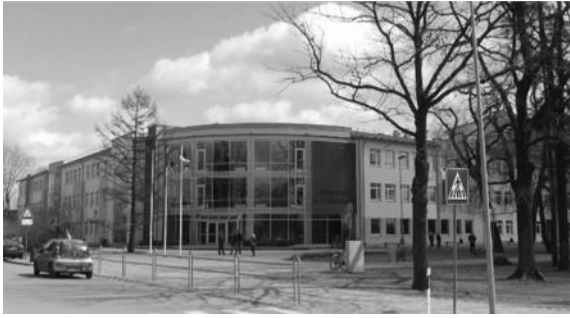
Fig. 1. Facades of Jelgava Secondary School No. 4 [Source: photo by author private archive, 2013]
