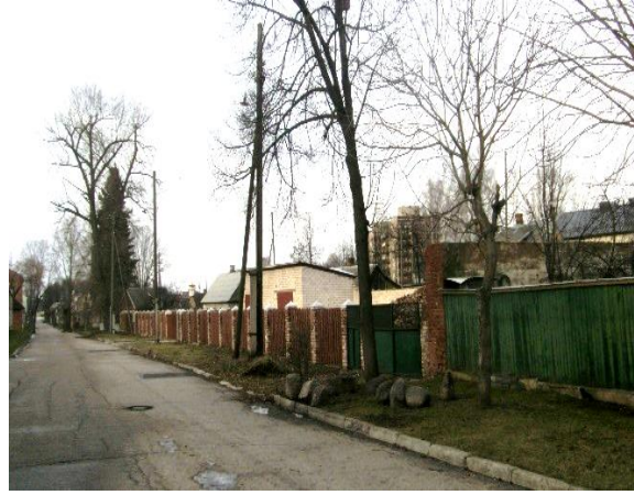
Fig. 10. Building on Vidus Street 31/33, January 2015 [Source: www.panoramio.com/user/420066? with_photo_id=32767610 ]
