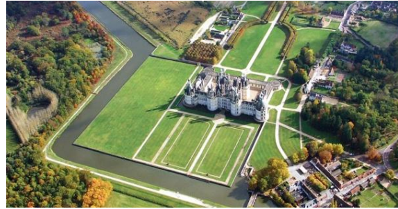
Fig. 5. Chambord Castle in France. The parking lot, restaurants and cafeterias are located in the nearest neighborhood [Source: http://www.lefigaro.fr/culture/2013/04/16/ ]
