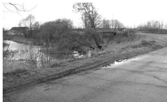
Fig. 1. The historical roadbed with an old wooden bridge over the river Platone [Source: photo by author, 2014].
