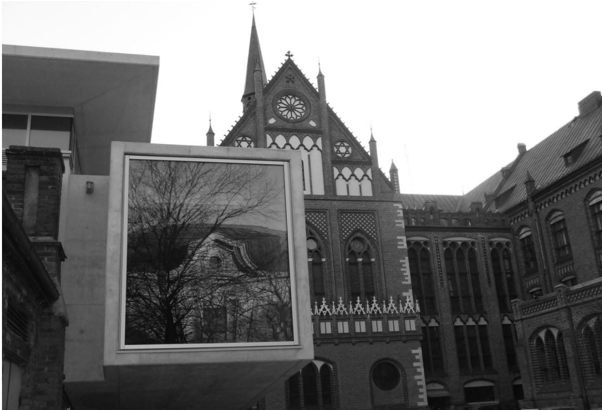
Fig. 1. New addition of the Art Academy of Latvia designed by SZK and partners. Facades, view from building's backyard [Source: photo from author's private archives].
