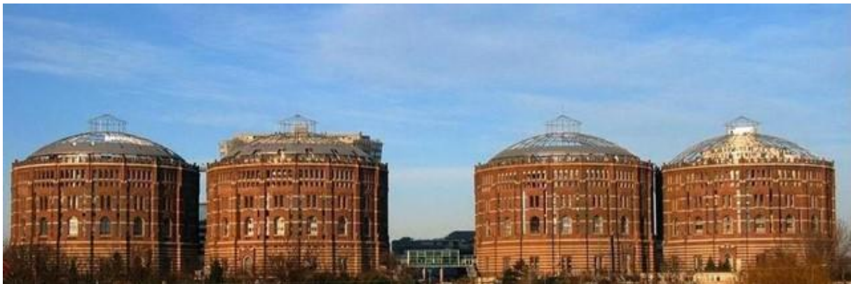
Fig. 2. Gasometer - a city within a city
